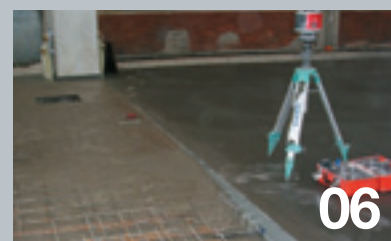
Concrete can be on both side of Ideal Joints at the same time or alternate days to separate two placements.
