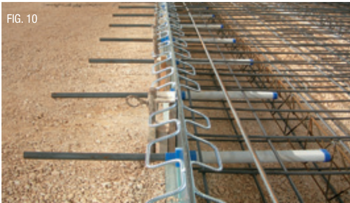
FIG. 10 Detail of Ideal Joint System® installed and ready for the concrete placement.
