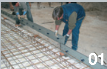
Positioning on the joint line.
