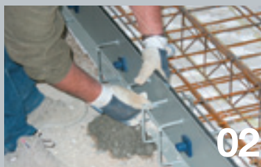
Installation with PVC screws.
