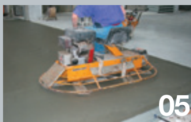
Finishing of the concrete slab.
