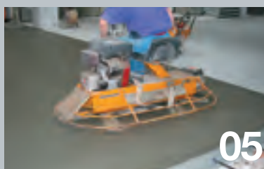
Finishing of the concrete slab.
