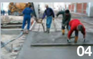
Concrete placement.
