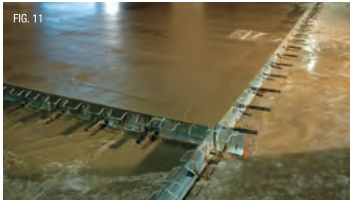
FIG. 11 Detail of Ideal Joint System® ready for the next placement of concrete.
