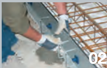
Installation with PVC screws.
