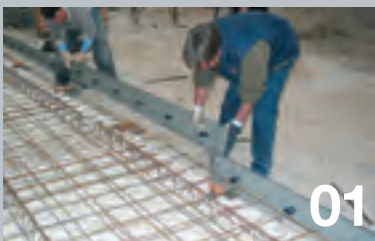
Positioning on the joint line.
