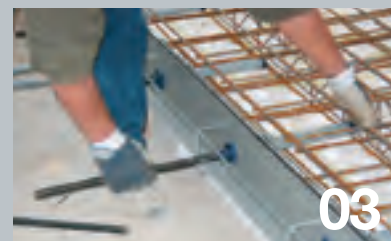
Installation of the plastic sleeves and dowel bars.
